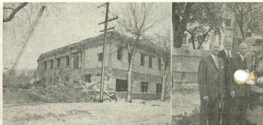
Our old Central TB Clinic was chosen as the site for the hospital. Demolition began in March, 1960. On June 6, 1960, staff and watch the Minister of Health.
