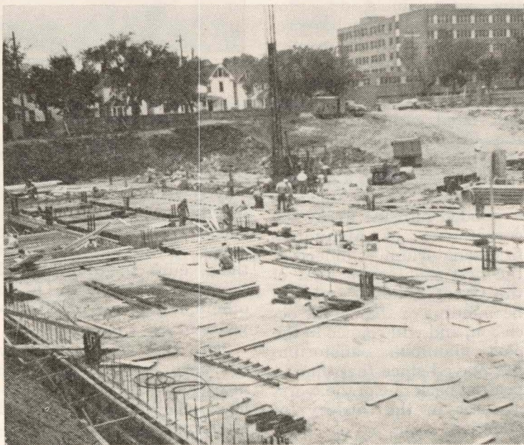
HOSPITAL BUILDING UNDER WAY—Sanatorium Board staff mem-
