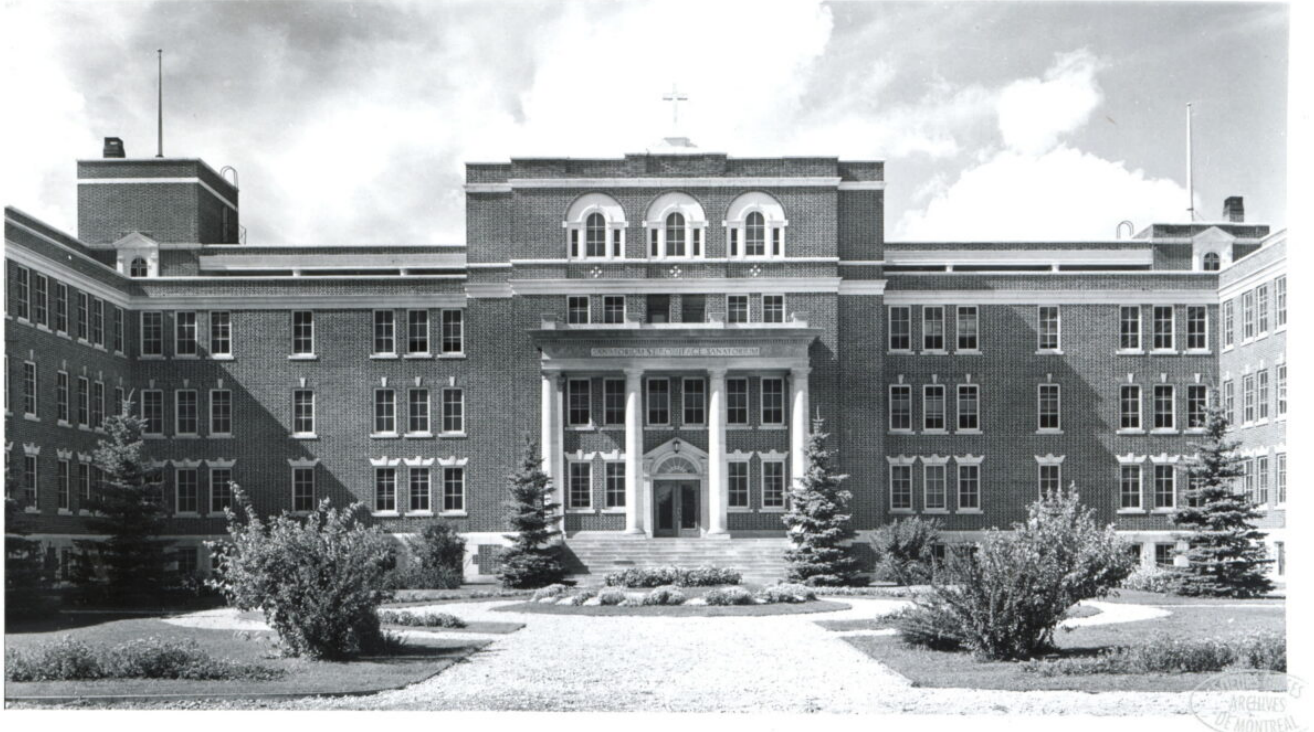
Main building, St. Boniface Sanatorium, Grey Nuns of Montreal, L098-Y1B
