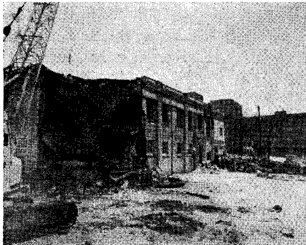
Demolition of the Central TB Clinic in March 1960.
